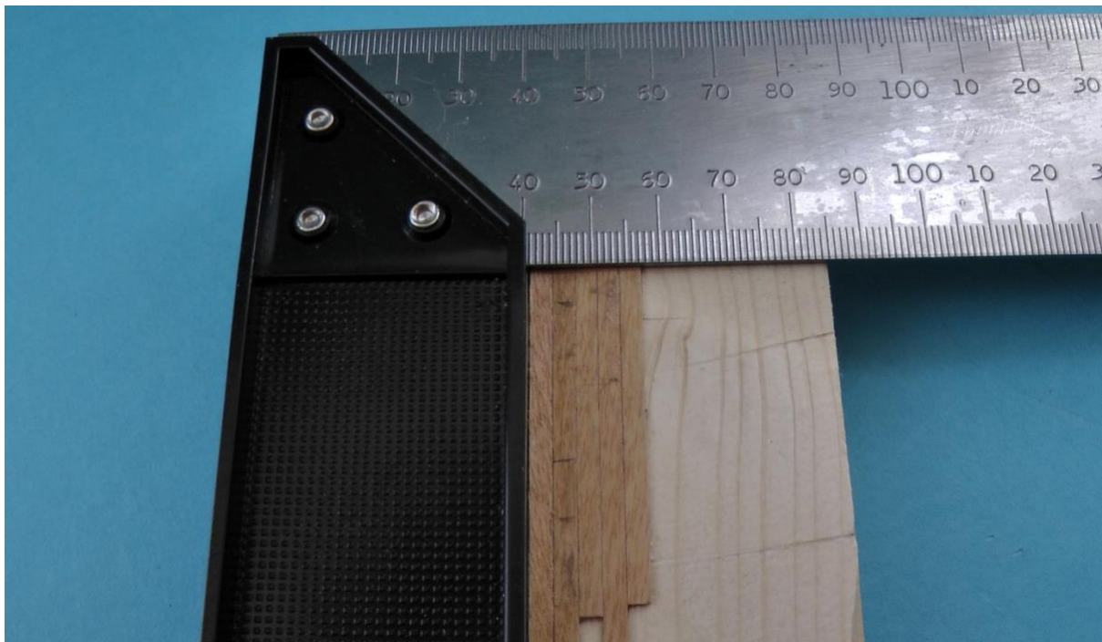
Figure N24 - Square line being drawn on the planks
